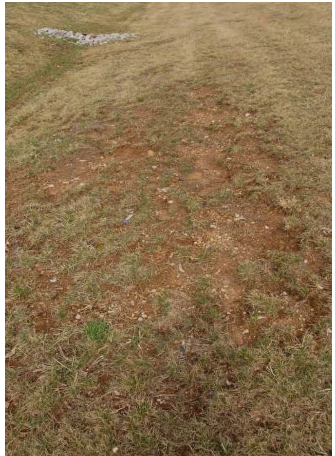
Erosion is present on the side slope of this grass swale.
