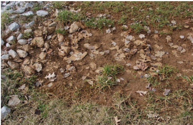
Evidence of sediment deposition next to riprap. Excess sediment reduces stormwater infiltration into the underdrain.
