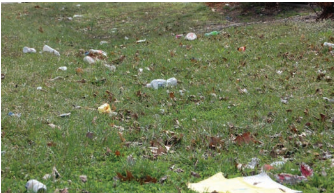
Trash and debris accumulate in a grass swale. Trash and debris should be removed after every rain of more than one inch.
